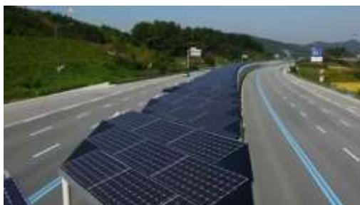
The South Koreans have taken a different approach by combining cycling and solar panels. When they designed a twenty mile long, six lane highway between the cities of Daejeon and Sejong, they incorporated a bike lane running down the center -
